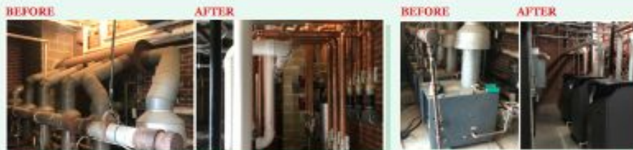
ST. MARY MAGDALEN BOILER REPLACEMENT
